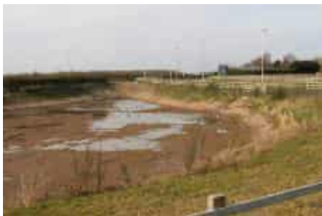
Attenuation pond/basin almost dry (Main Site)
