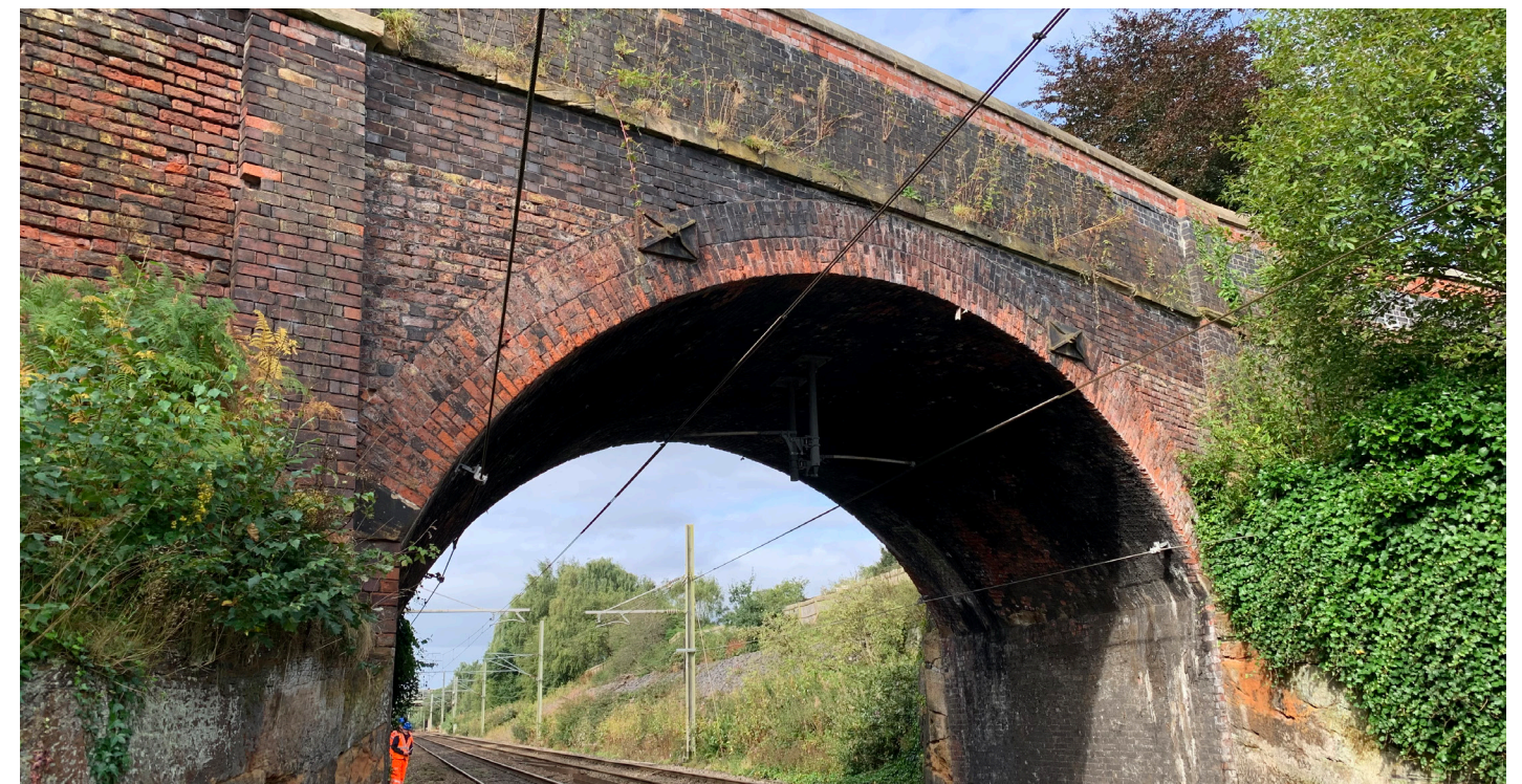
Figure 3.17 Parkside Road Bridge viewed from the south looking west September 2024
