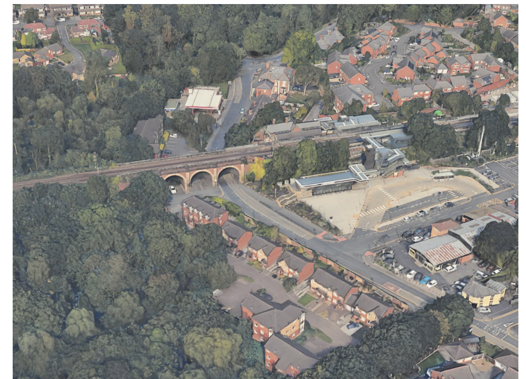
Figure 3.42 View of the viaduct and station showing the setting September 2024
