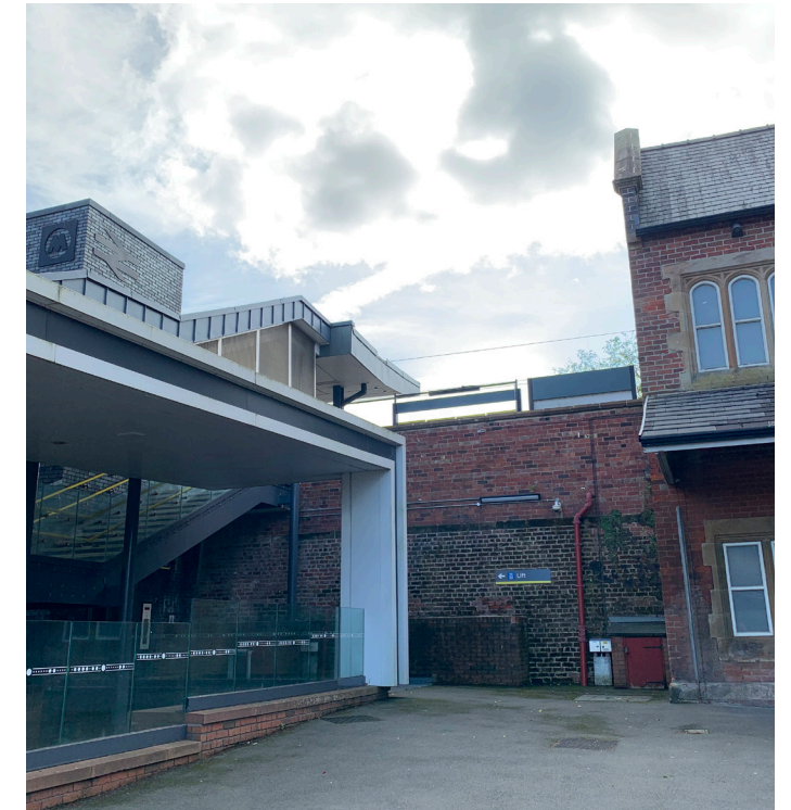
Figure 3.40 Modern extension on Newton-le-Willows Station September 2024
