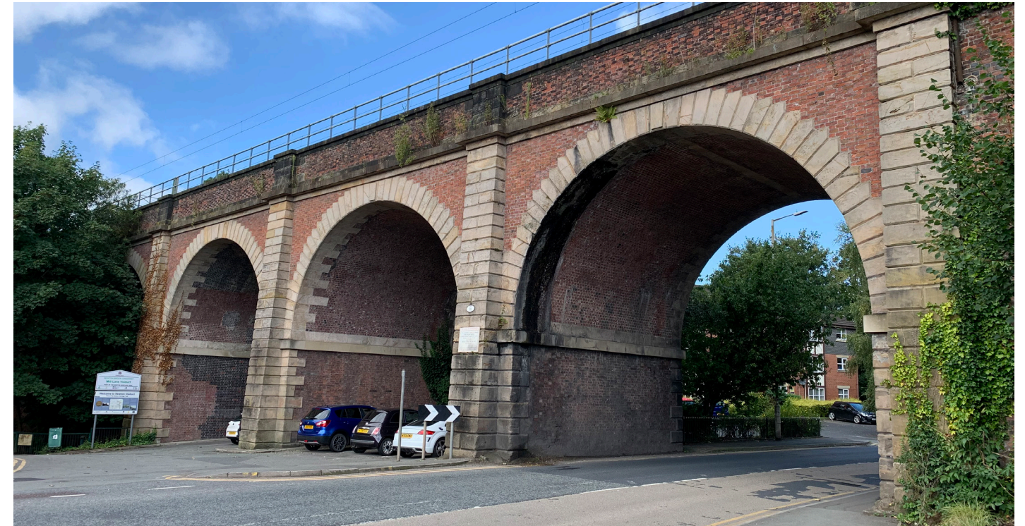
Figure 3.43 Newton Viaduct to West of Station September 2024
