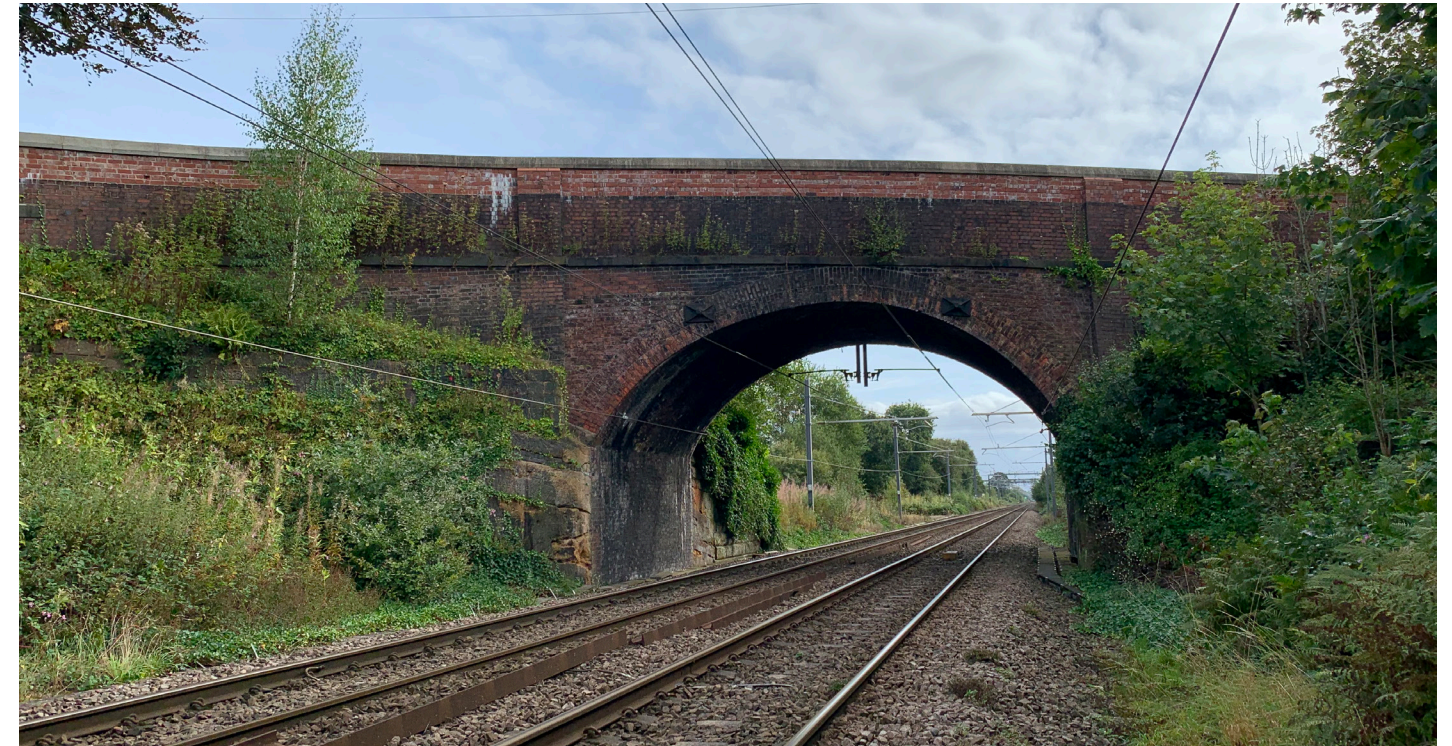
Figure 3.16 Parkside Road Bridge looking west September 2024
