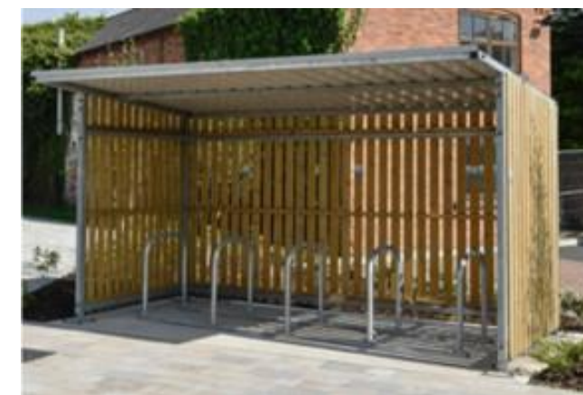
Fig 29. Illustrative Sedum roofed and timber clad cycle shelter
