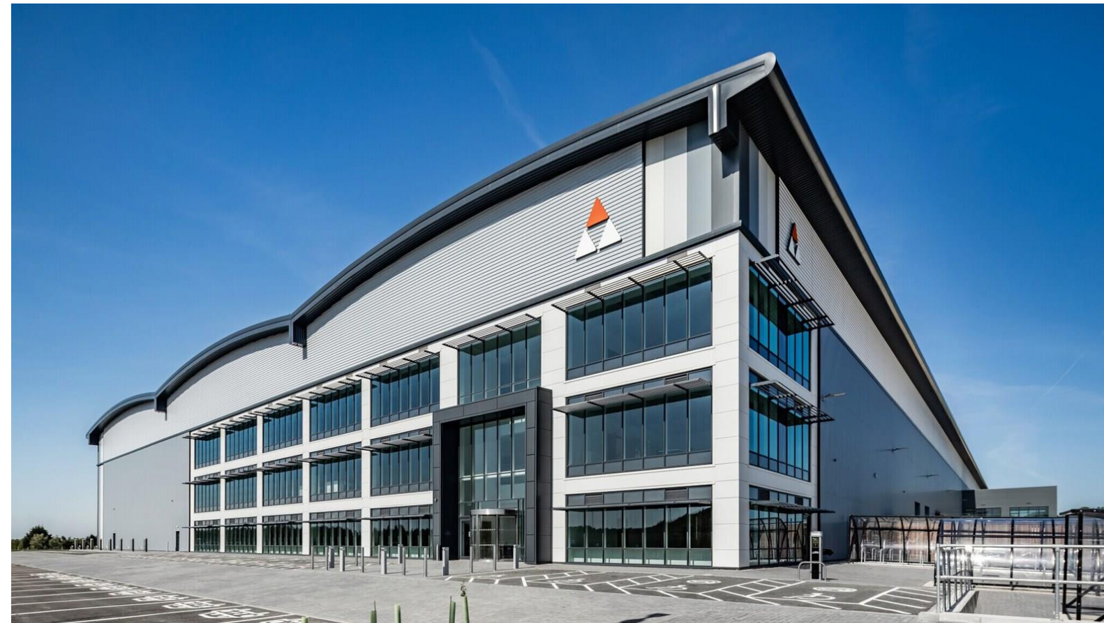
Fig 22. Illustrative Facility and Consistent Application of Materials and Colours
