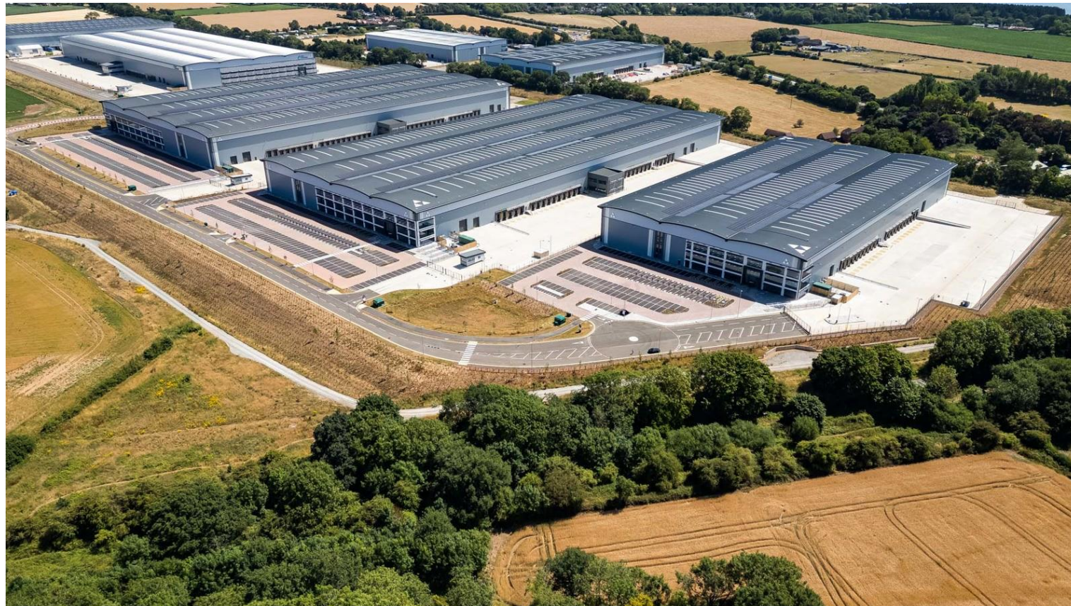
Fig 23. Aerial Image of a TBB development illustrating a consistency of design approach.
