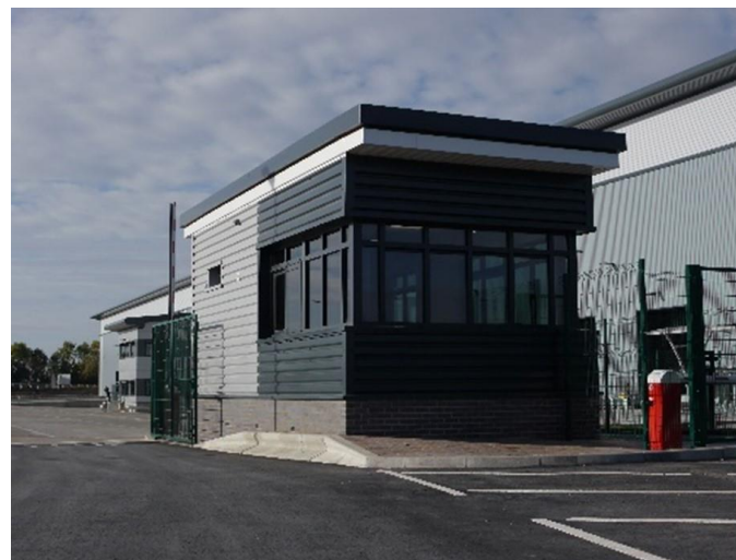
Fig 31. Example of secure gatehouse at entrance to service areas
